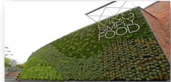
Marks & Spencer, Ecclesall Road, Sheffield, UK
